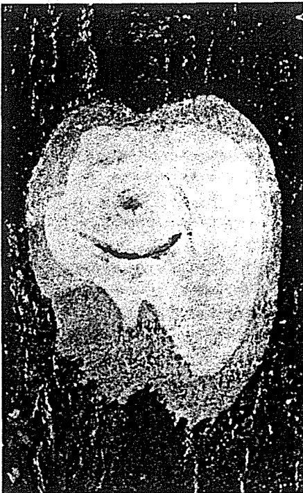
Figure 3. Flush cut branch on a young oak. Flush cuts covered with wound dressing have been the recommendation for pruning for over a century. There are no scientific data to support benefits of such treatments.
